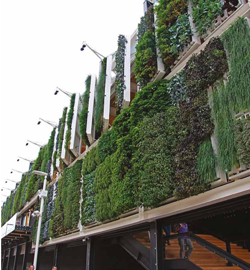
Figure 5. Kinetic green façade for sustainable food production. American Food 2.0 at Expo Milan (2015) by James Biber. Photo: B. Widera.
