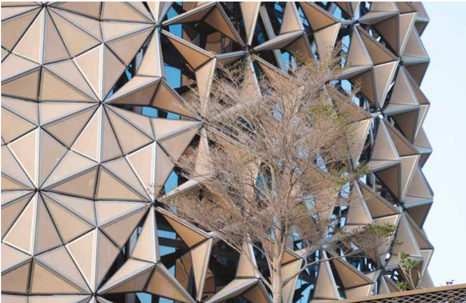
Figure 3. Kinetic façade system in Al Bahar Towers (2012), Abu Dhabi by Aedas Architects. Photo: B. Widera.
